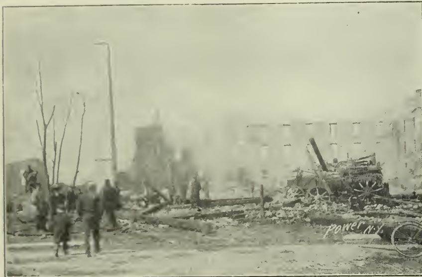
FIG. 1. SITE OF BOILER ROOM, AT BASE OF STACK
